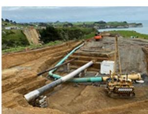
Firstgas is making good progress on its Gilbert Stream realignment project to increase the resilience of the Maui pipeline transmission network. The \$13 million project near Pukearuhe, 50km north of Taranaki, involves moving 370 metres of high-pressure gas pipeline inland because of the risk by cliff erosion.
